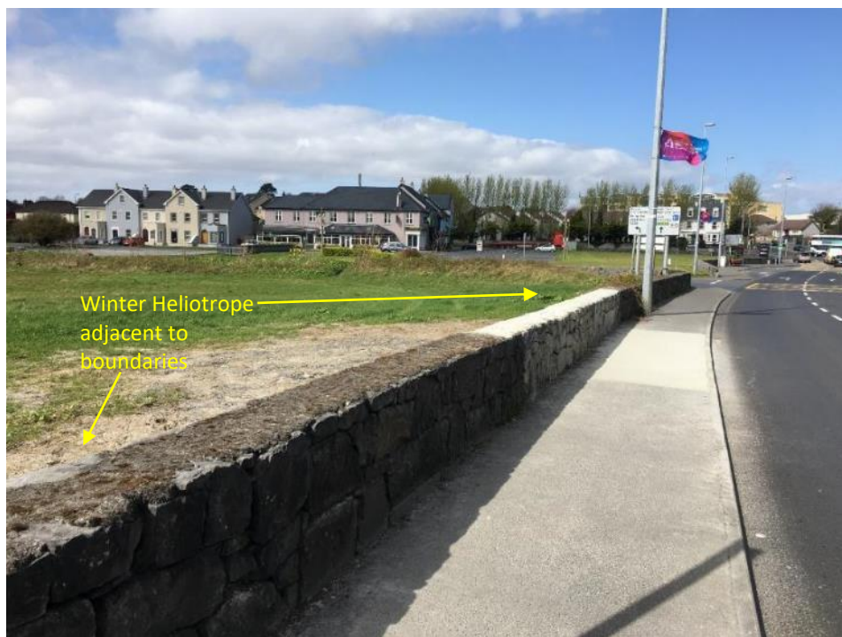
Photo 6. Showing the approach to Moneenageisha junction on the Dublin Road. Note the disturbed ground and wall repairs.
