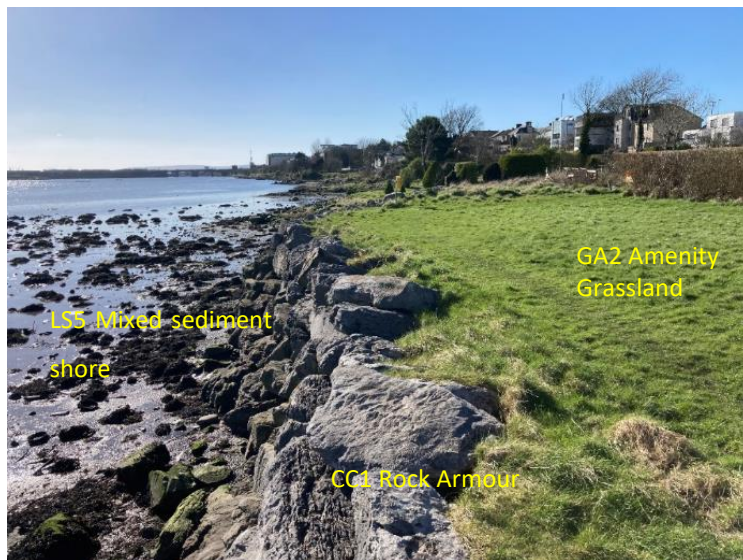
Photo 5. Showing the habitat types at Lough Atalia Playground and adjacent amenity grassland adjacent to Lough Atalia.
